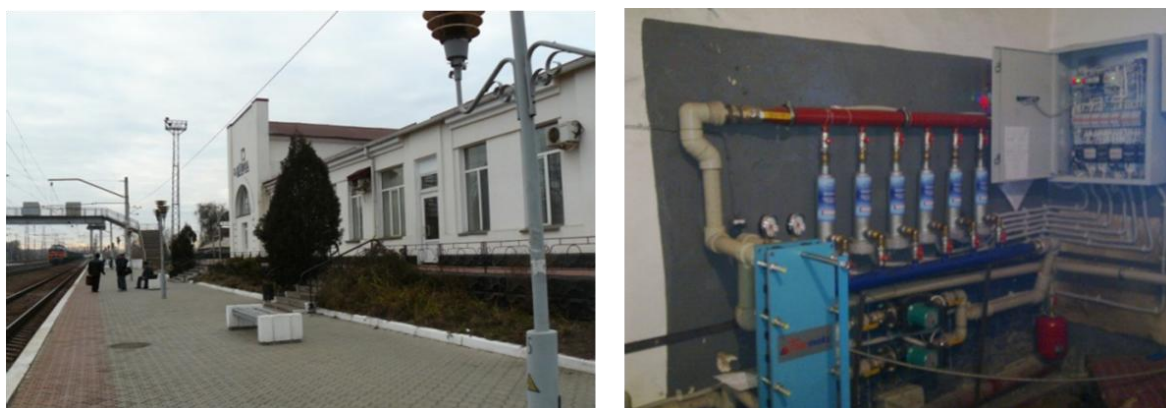
Fig. 3. Premises Station, Station Diyivka
