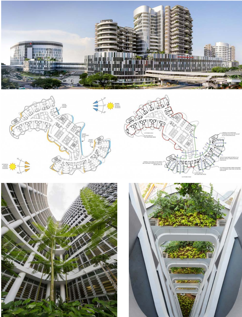
Figure 1. Bioclimatic facade system in Ng Teng Fong (NTFGH) i Jurong (JCH) Hospital, CPG Corporation, Singapore, 2015
