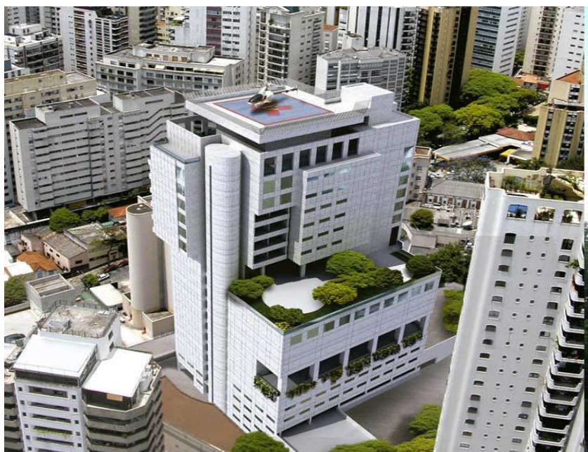
Figure 5. Bioclimatic facade system in Samarito Hospital, Brazil, 2009
