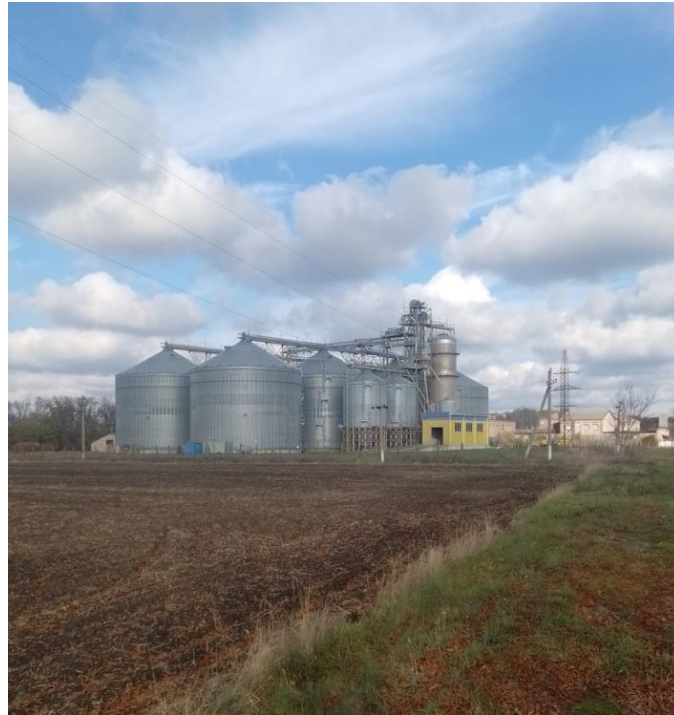
Figure 2.2 – Silo structures with flat concrete bottoms
