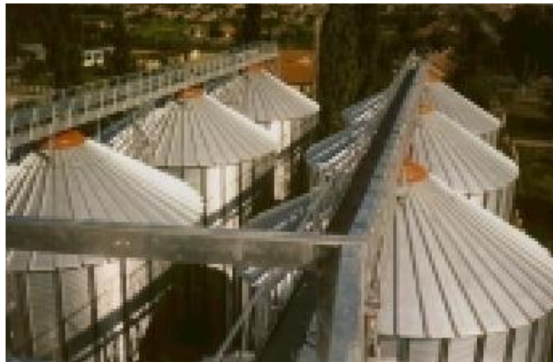
Figure 2.3 – Galvanized steel silo blocks
