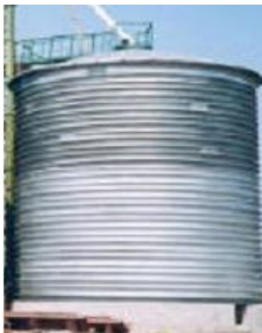
Figure 2.4 – Spiral-wound silo with folded joints
